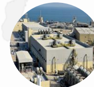
Al Khobar I desalination plant Saudi Arabia
